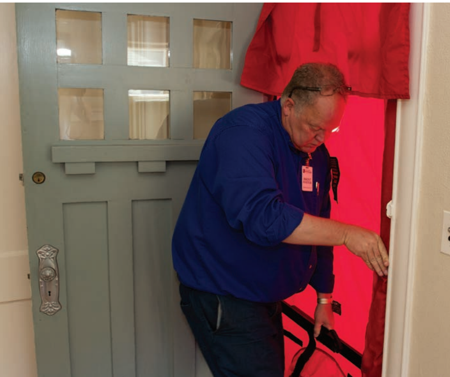
Setting up a blower door.
